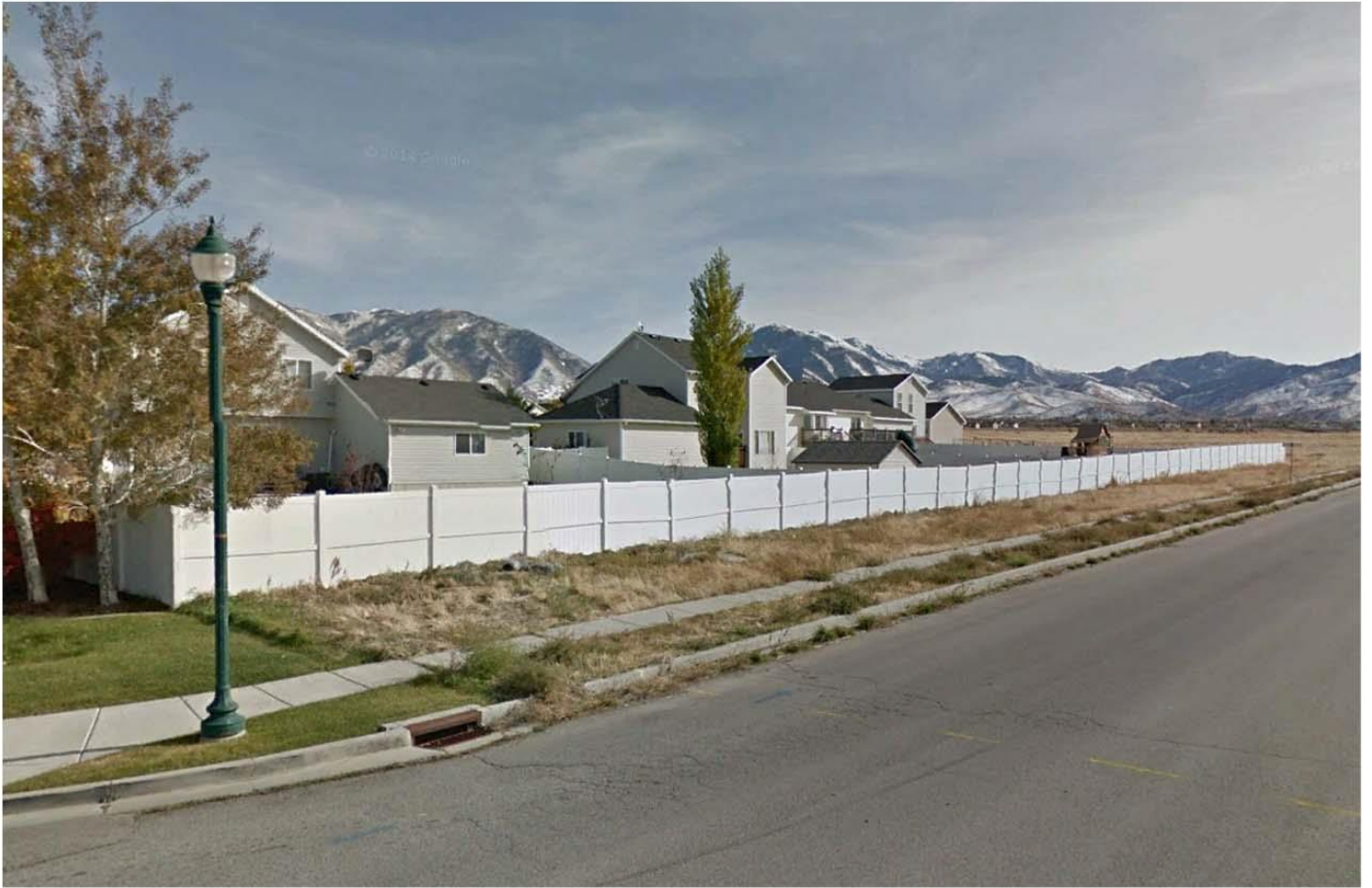
Existing 400 West Fencing
